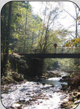
Fish Dam Creek Bridge
